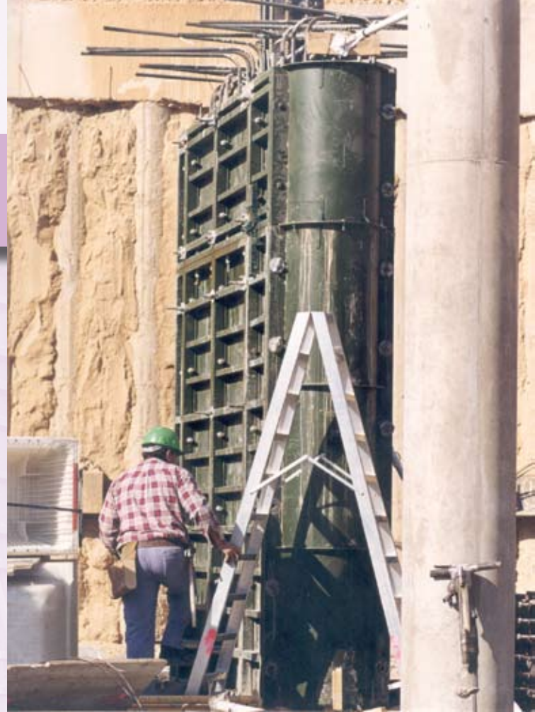
oval pillar with heavy range wall screens and heavy range round formwork
